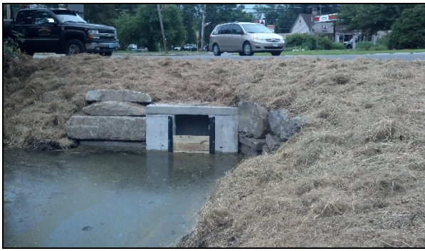
New drainage culvert, inlet structure and headwall at Rotary.
