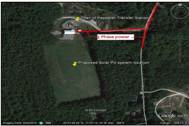
Aerial image of the proposed PV Solar project site.
