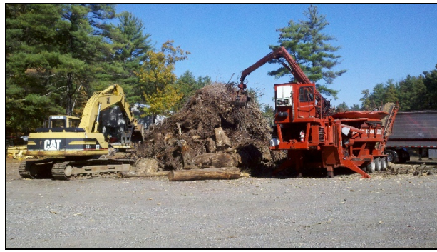
Stockpiled storm debris being processed and removed from Highway yard.
