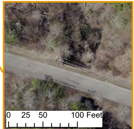
Heald Street Culvert 42.670185, -71.613507
